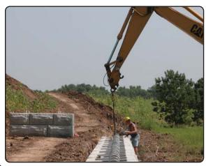
prior to placement of leveling pad materials. The contractor shall replace any unsuitable soils discovered during excavation at the direction of the engineer.
